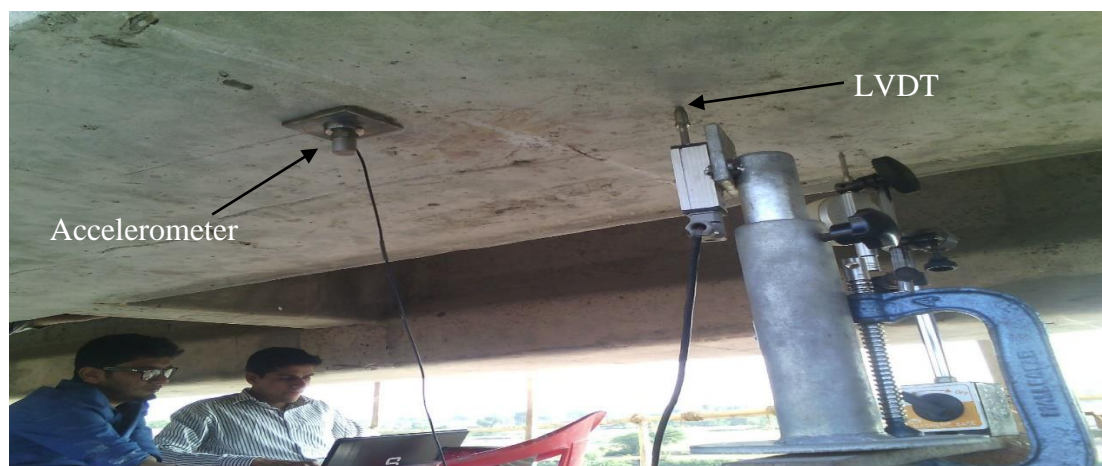
Fig 2. Structural health monitoring of Ratlam railway bridge with help of sensor
